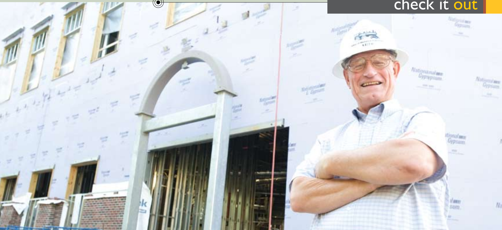
Hawks' Eye: Keith Hawks, professor and assistant head of mechanical engineering, before the rising wing of the Mechanical Engineering Building. (Photo by Andrew Hancock)
